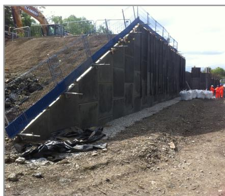
Reinforced Earth Co. Ltd (RECo) was employed to design and supply the components for Muller Road Reinforced Earth retaining wall, as part of Network Rail's upgrade plan to increase the rail capacity from two tracks to four tracks between Dr Day's junction to Filton Abbey Wood, to the north of Bristol.
