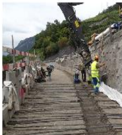
Friction Link system with synthetic strips
