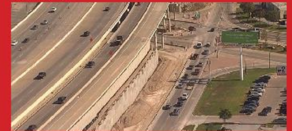
North Tarrant Express near Dallas, Texas, USA
