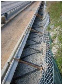
Direct Link system with synthetic strips
