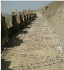
Friction Link system with steel strips
