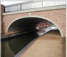
As part of this project, a new canal bridge was required to replace an existing masonry structure. The conforming scheme for the bridge comprised of a simple supported single span deck on piled abutments.
